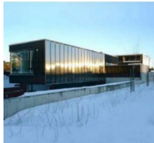
Figure 6: Using solar panels in the façade [12]
