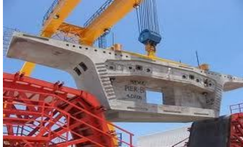
Figure 5. Precast component to be installed in precast type of bridge
