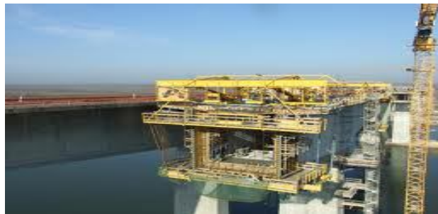
Figure 6. The structure of in-situbalanced cantilever
