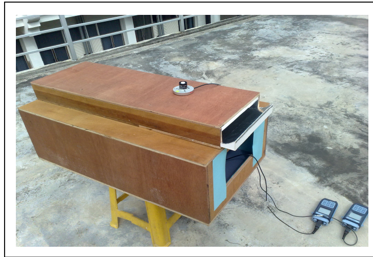
Figure 1. Construction and Installation of scale physical model on selected site
