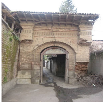
Figure2.6. Entrance of a private alley in an old neighborhood in which underlying structures of the roof are made of wood, Babol, Mazandaran, Iran.
