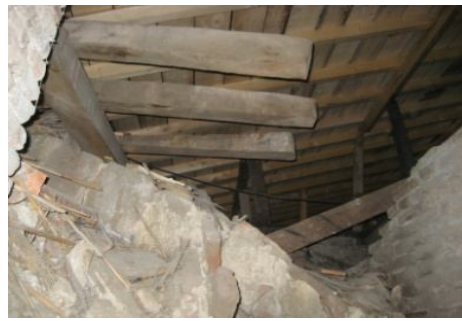
Figure2.11. Application of wooden ladders for establishing the roof on the top of mosque entrance.
