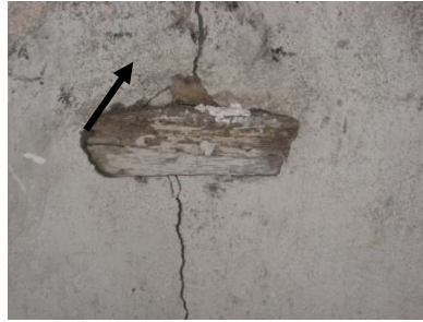
Figure2.7. A wooden beam which is crossed from inside the wall of staircase and connected to minarets and roof.
