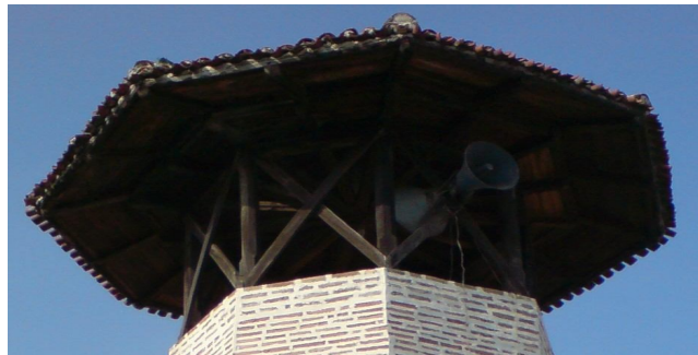
Figure2.5. Minaret of Imam Hassan Askari's mosque where top of the minaret is a wooden structure, Amol, Mazandaran, Iran.
