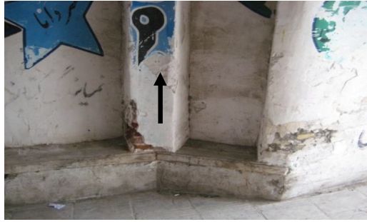
Figure2.16. A sitting place for the old in Hami passage where columns are based on wood, Sari, Mazandaran, Iran.
