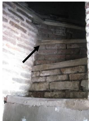
Figure2.13. Application of wood in the end of bricklaying of stairs
