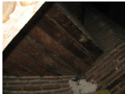
Figure2.10. Application of planks in staircase roof connected to the roof area.
