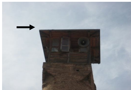
Figure2.14. Top of the minaret above the entrance of mosque which is made of wood.
