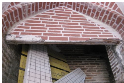
Figure2.12. Application of wood in staircase connecting to the roof area
