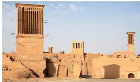
Figure 7. Four-sided windcatcher (Reference: authors' archive)
