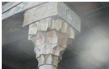
Figure 2.6. A picture of a square head pillar and painted wooden mogharnas in Firozkala sanctuary- Amol
