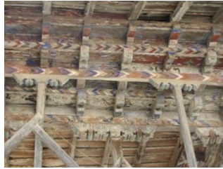
Figure 2.3. A view of pillar, its head (Kamacheh), nal, edge strap, vavand, shirsar, flaring, hala (from silk wood), board and seamless flooring in Pasha sqatar of Kala-Amol
