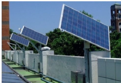
Fig.3. installing tracker system on buildings
