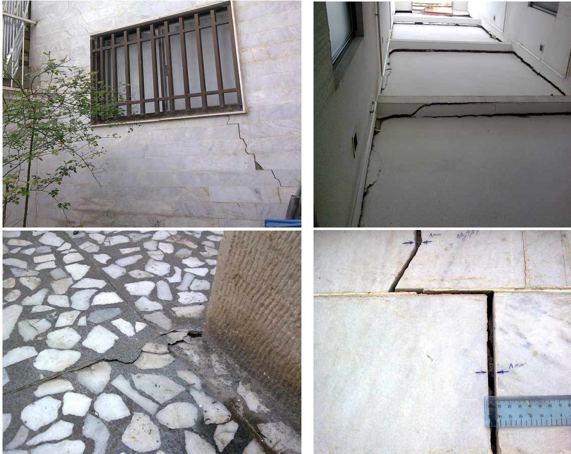
Figure 8. cracks in different parts of the old building due to adjacent building construction
