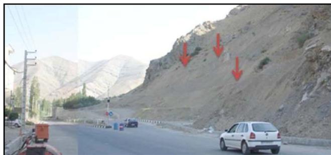
Fig. 13: Rotational slide in debris Haji Abad -Oshan Road (one km to Oshan), the instigation of susceptible mass (raining and previous landslide)With road construction activity (view to north east).
