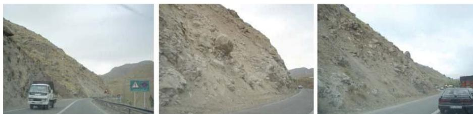
Fig. 14: Landslide in rocks and debris on unstable slope in Abali – Amol road (View to north).
