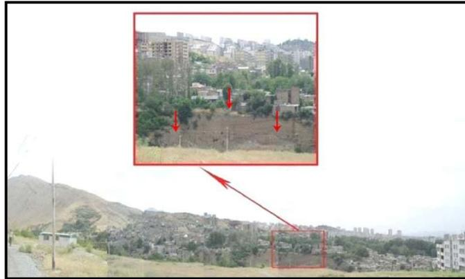
Fig. 15: A view of rotational slide in debris in Shahrak Majles region (view to north east) .
