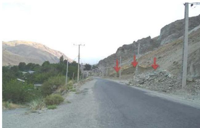
Fig. 17: landslides of road around of Latyan Dam (in right hand falling)
