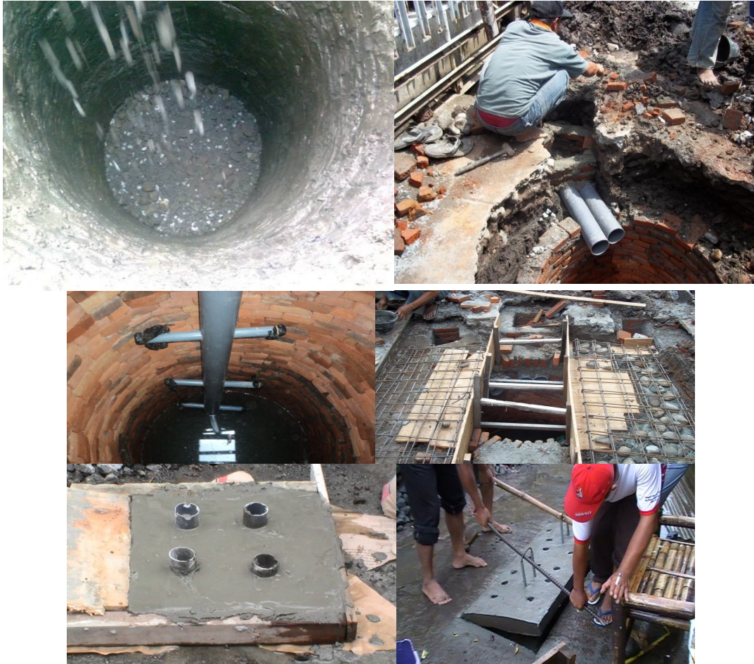
Figure 4 Finishing work. (a) Installing stairs. (b) Making well cover
