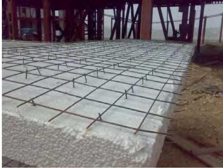
Fig 1. Different Parts of Sandwich Panels
