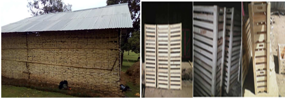
Figure 1: The house constructed above underground pit and wooden box used inside the storage to hold fruits
