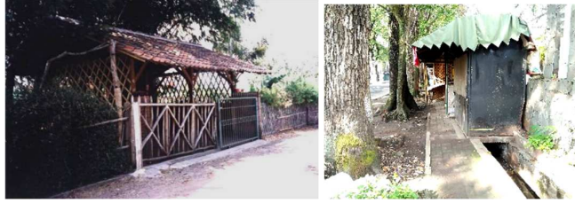
Figure 6 : Private Control To The Green Belt (a) and Drainage (b) Through Temporary Intervention
