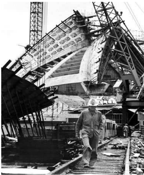
Image No. 3: manner of structural execution of complex
