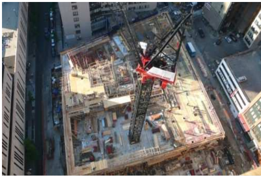
Image No. 22: view of concrete structure progression of Beekman tower
